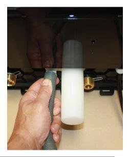
Figure 17: Condensate trap installation
