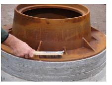
1 Clean and dry the flange of the casting frame and the top 4-inches of the cone section, with a wire brush and a whisk broom or rag.
