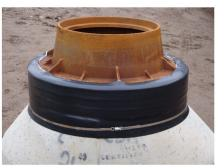
**5** Install Stainless Steel band at bottom of sleeve with 5/16" nut driver.
