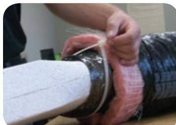
Secure the vinyl duct to the insulated transitions portion using the provided tie wraps.
