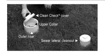
The following steps will guide your plumber through a proper inspection of your Clean Check® Extendable Backwater Valve.
